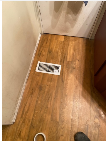
4. Bathroom floor, first layer. No asbestos detected.
