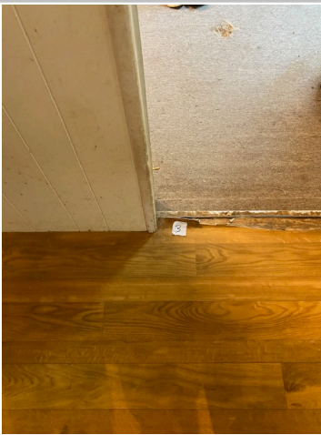
3. hallway floor, first layer. No asbestos detected.
